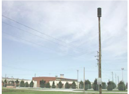
Base alert warning system.
