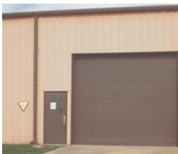
Mark contaminated buildings.
