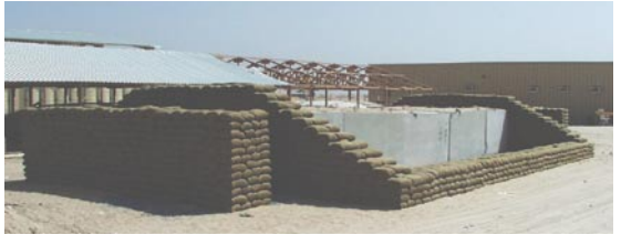
Semi-hardened bunker, without collective protection.
