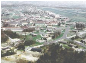
The airbase consolidates contaminated waste.
